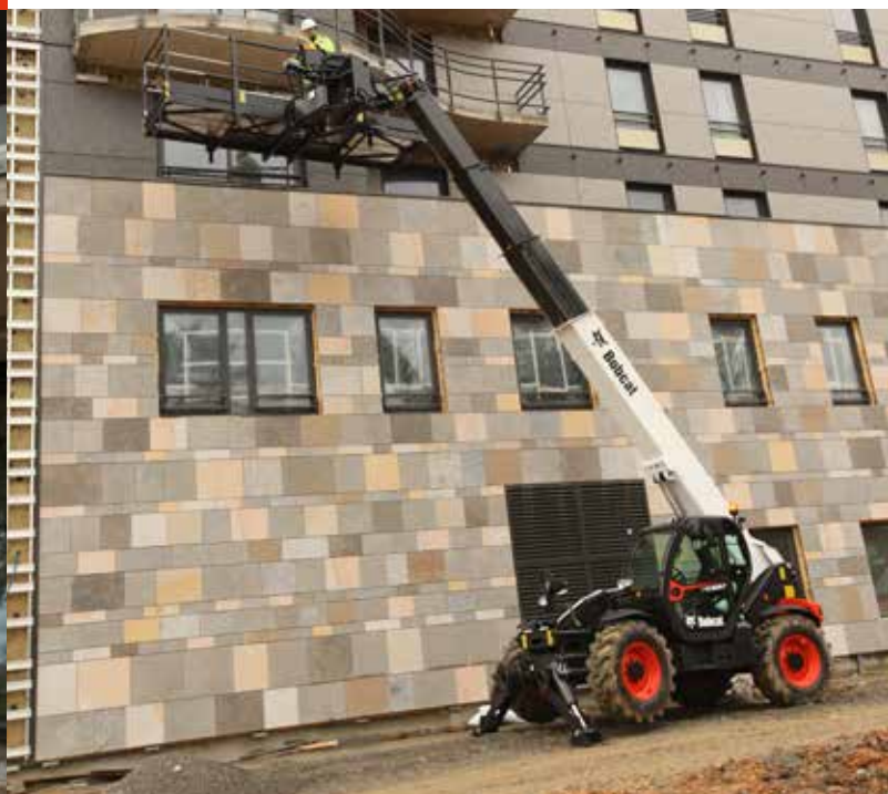
Man-platform: can be fixed, rotating and/or extendable
